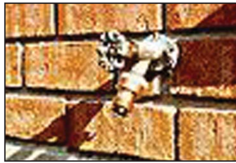
Figure 9.17. Hose Bib With Vacuum Breaker
