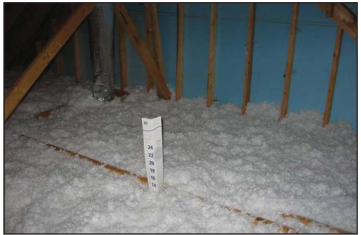
Figure 7.3. Depth of Attic Insulation
