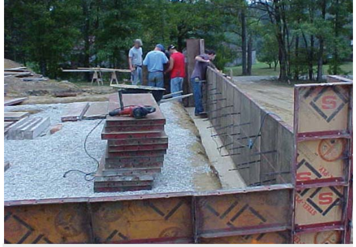
C. Concrete will be poured into this form on top of the footer to create the foundation of the home. Again, reinforcing rods are added to ensure that the concrete has both lateral strength, as well as the strength to support the home. Once the concrete has hardened and becomes seasoned, the forms will be removed to reveal the finished poured concrete foundation over the perforated drainage pipe. Not shown is a newer technique of using insulating polystyrene forms and ties in a building foundation.
