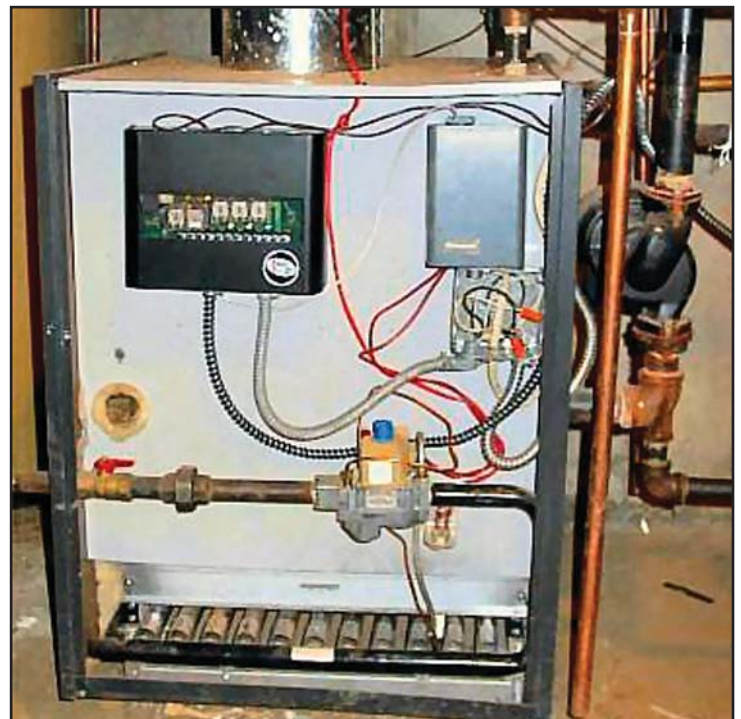
Figure 12.9. Gas-fired Boiler
