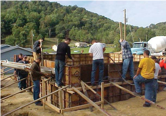
D. Foundations are not always poured concrete, but are often cinderblock or similar materials that are cemented in place to form the load-bearing wall. The arrow shows the concrete chute delivering concrete into the form. Long poles are pushed into the freshly poured concrete to remove air pockets that would weaken the foundation.
