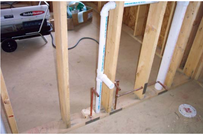
C. Vent for the sink and toilet, soil pipe, and cap for toilet connection shown. A wax or plastic seal shaped like a donut will be placed on the cap before bolting down the toilet.
