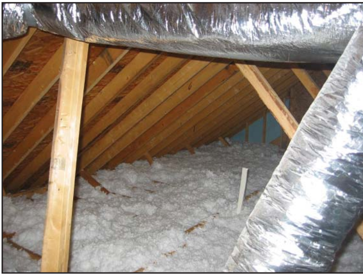
Figure 7.2. Blown Attic Insulation
