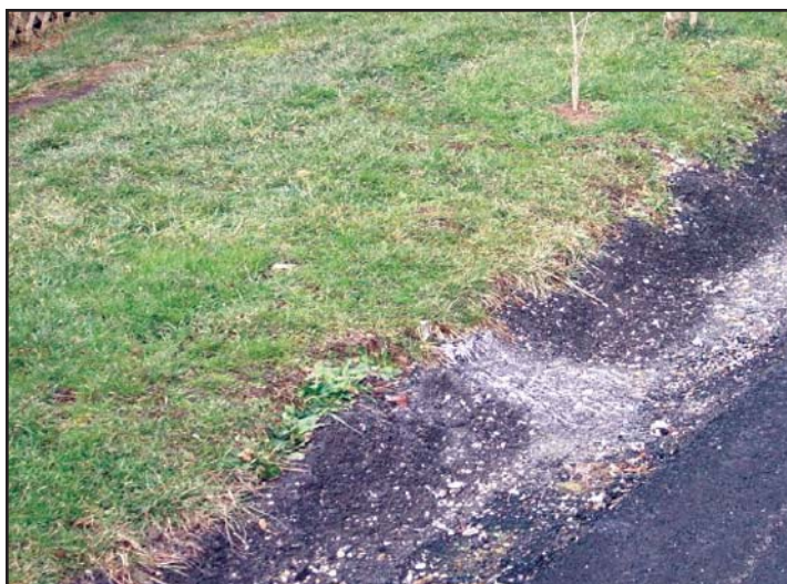
Figure 8.8. Sewage in Drainage Ditch
